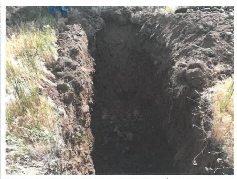
Photo 2 – Test Pit showing soil profile
